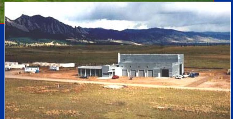
Industrial User Facility
